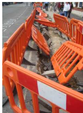
High Street pavement repairs in progress
